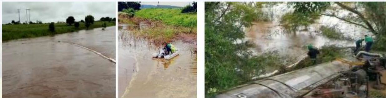
Heavy Rainfall and flooded river resulted in initial booming challenges, some diesel spilt downstream and deposited onto river banks in low flow areas
